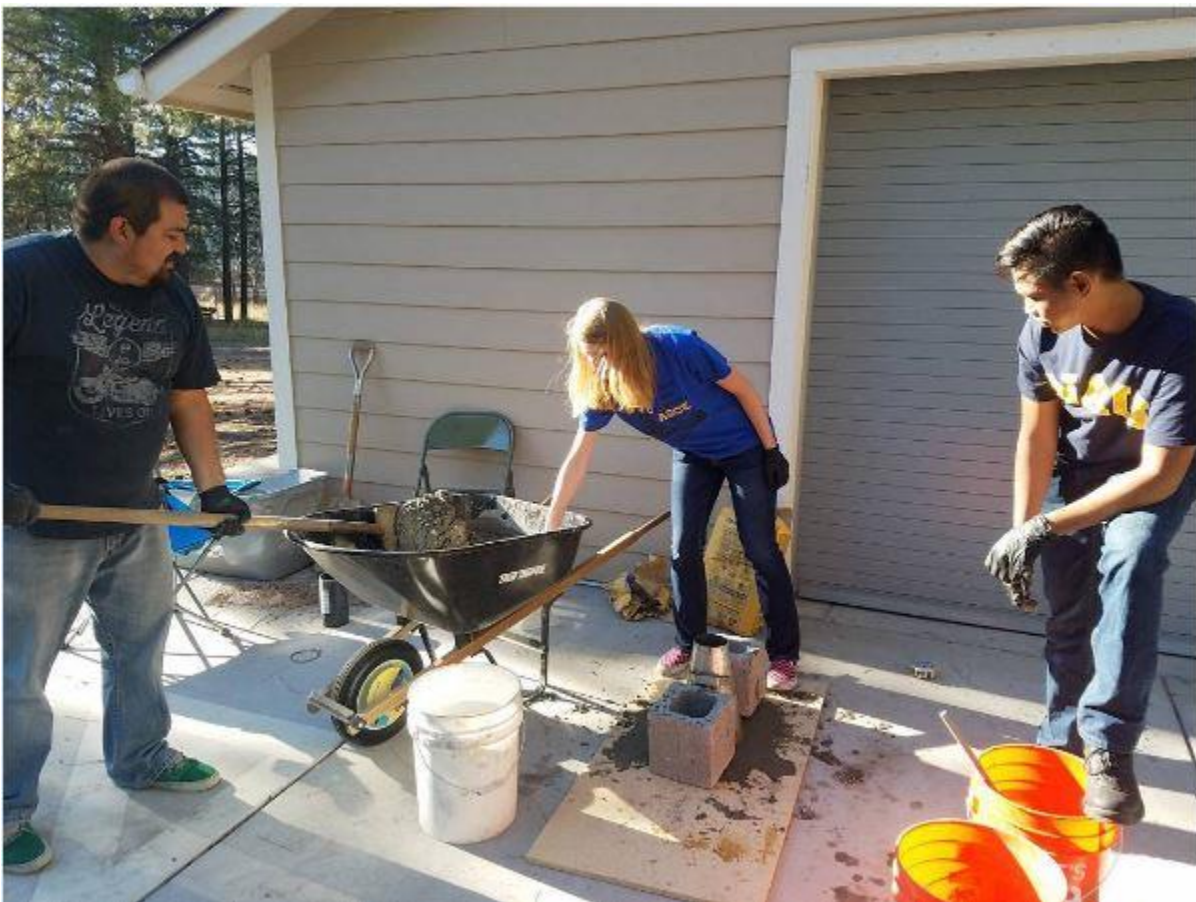
PHOTO 2 – Testing the slump of initial baseline batch mix
