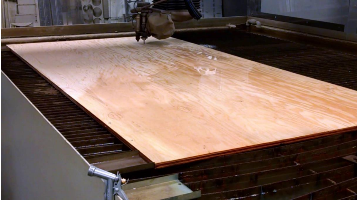
PHOTO 1 – WaterJet cutting of the cross sections by third party
