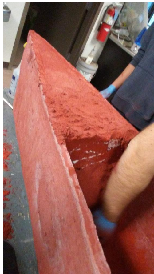
PHOTO 2 – Overlaying floatation with finishing mix
