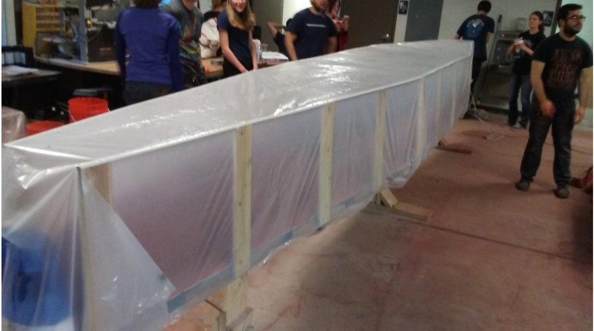
PHOTO 6 – Constructed curing chamber with two humidifiers at opposite ends
