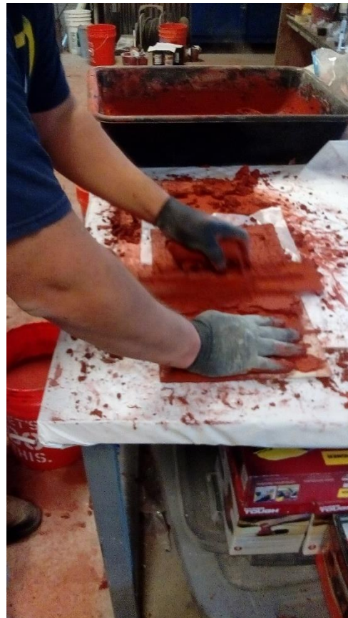
PHOTO 2 – Finishing mix strike off on the 1/8" tile molds
