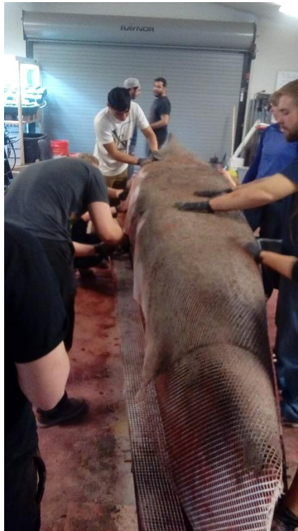
PHOTO 4 – Application of structural mix over mesh placement
