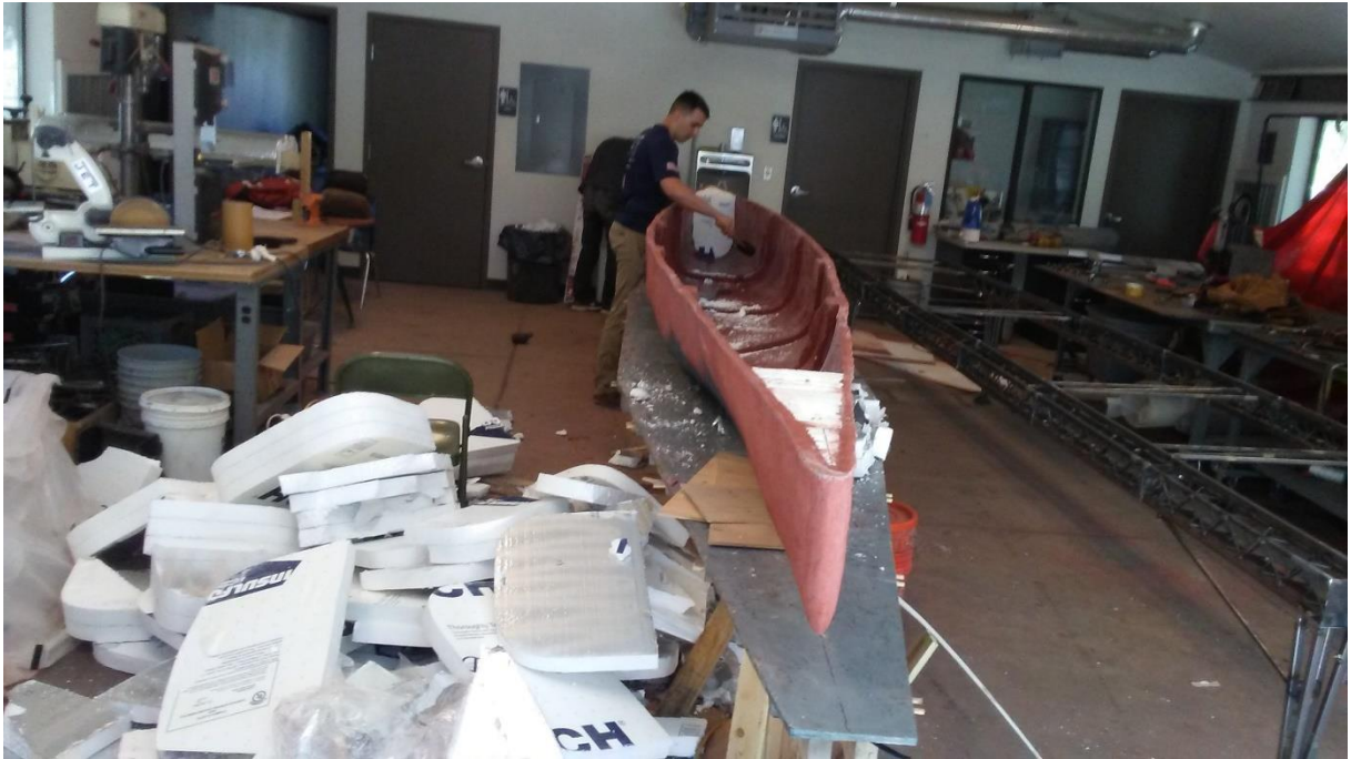
PHOTO 1 – Preparing to overlay end cap floatation with finishing mix
